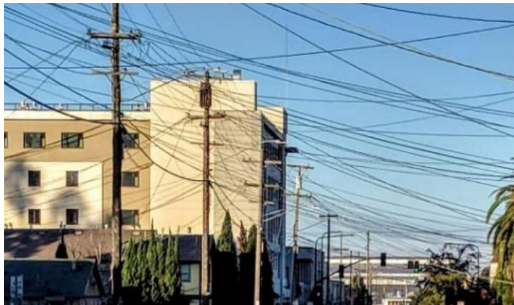
Dangerous overhead wires
