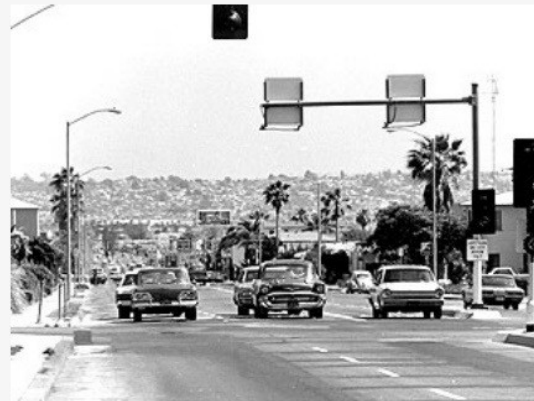
Mission Boulevard, circa 1972 - After Undergrounding
