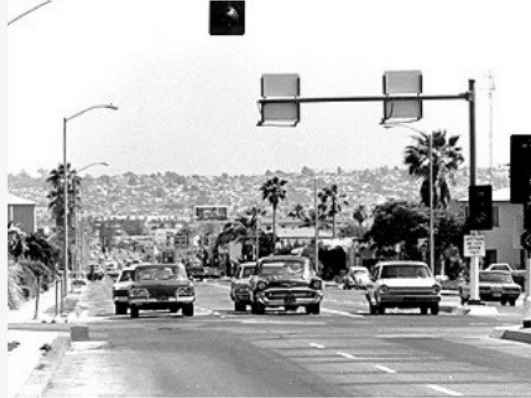
Mission Boulevard, circa 1972 - After Undergrounding
